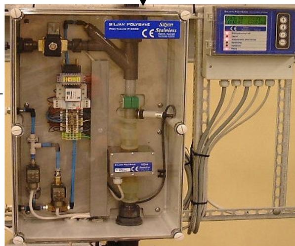
Indirect control of the DS-content of sludge from thickener
